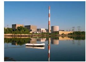
Millstone Nuclear Power Plant, Waterford, CT
